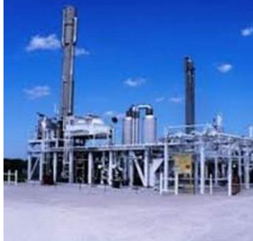
Natural Gas Processing Plant
